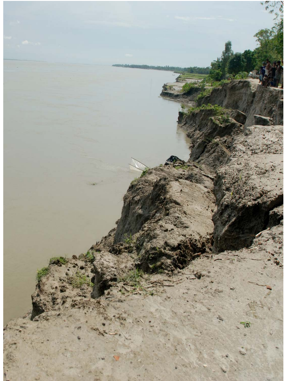
Riverbank erosion is already displacing hundreds of family everyday in Bangladesh as their homestead is washed away and claimed by the river current.
